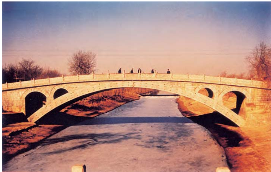
Zhaozhou Bridge in Hebei, built in the Sui Dynasty, is the earliest, well-preserved, single-arch stone bridge in the world.
