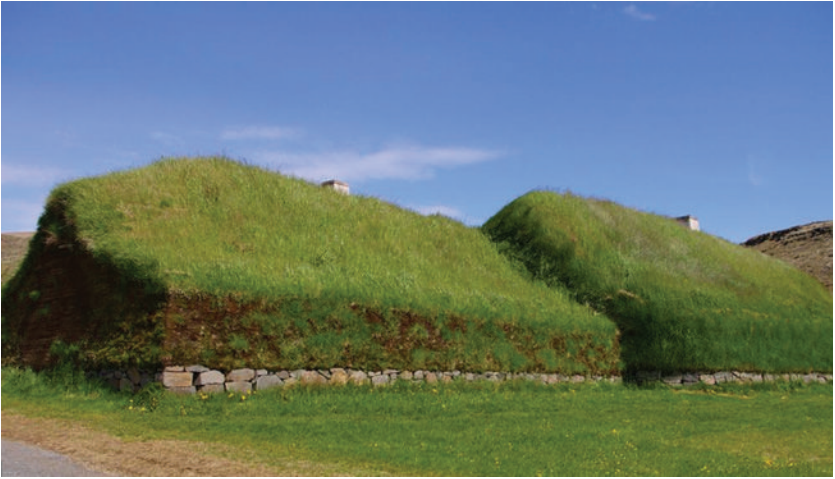
Figure 5. Photo of reconstructed Norse-style turf house in Iceland. Similar sod house construction techniques were brought to North America by Scandinavian immigrants in the 19th century (photo by Erik Erlandson).
