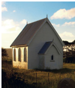
Simple, unadorned buildings, such as this one in New Zealand, characterize Baptist chapels.
